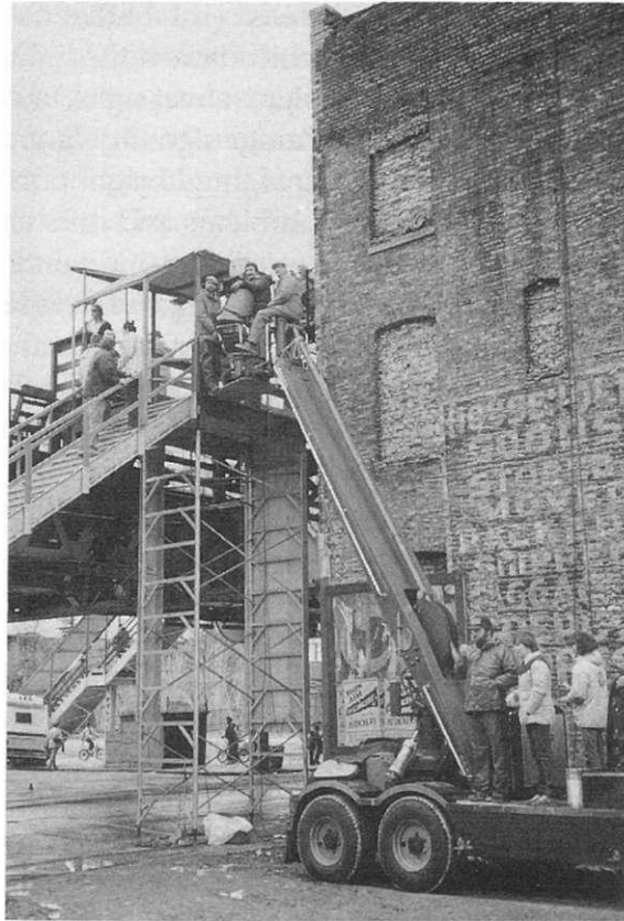
Figure 4.1 On the crane at the Chicago el station
