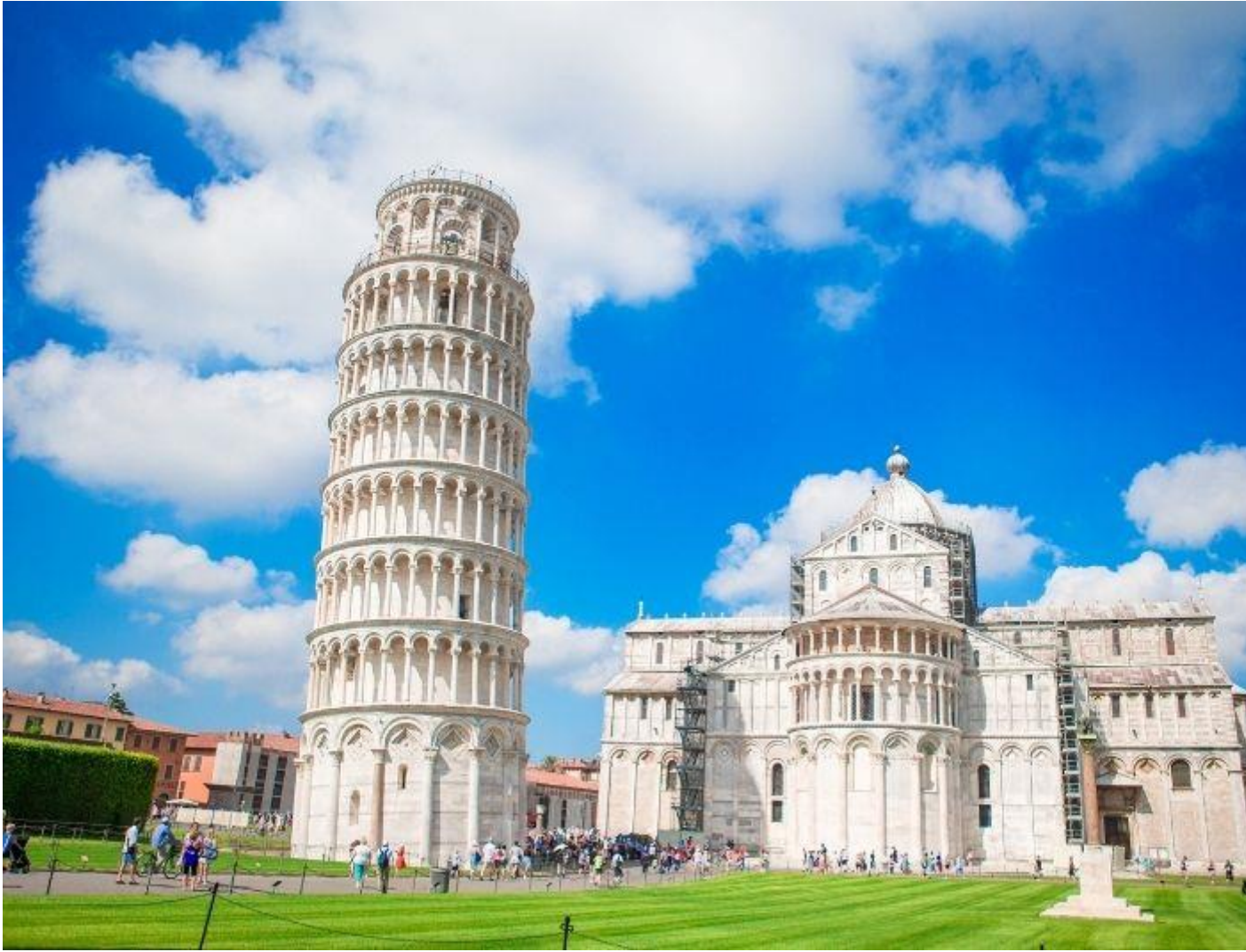
Leaning Tower of Pisa
